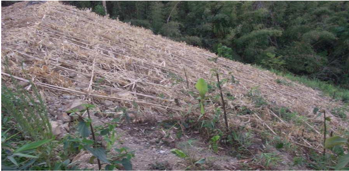
Figure 8-2 Bamboo Net Plantation
