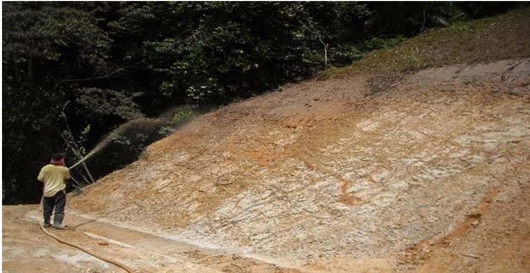
Figure 8-3 Hydroseeding
